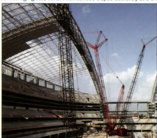
New Stadium Construction – Spring of 2008
